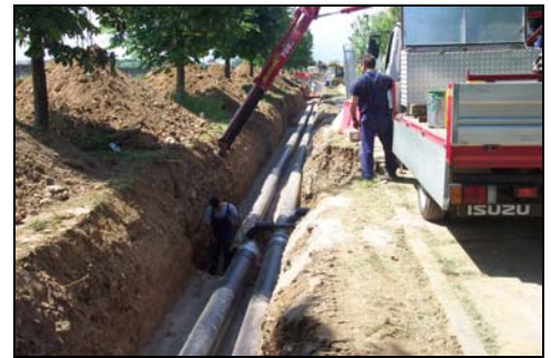
Workers laying a main trunk of the network.
